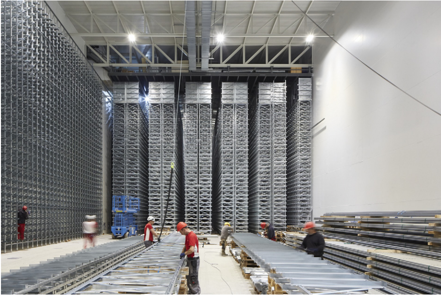
Constructing the high bay storage area © Ulrich Niederer
