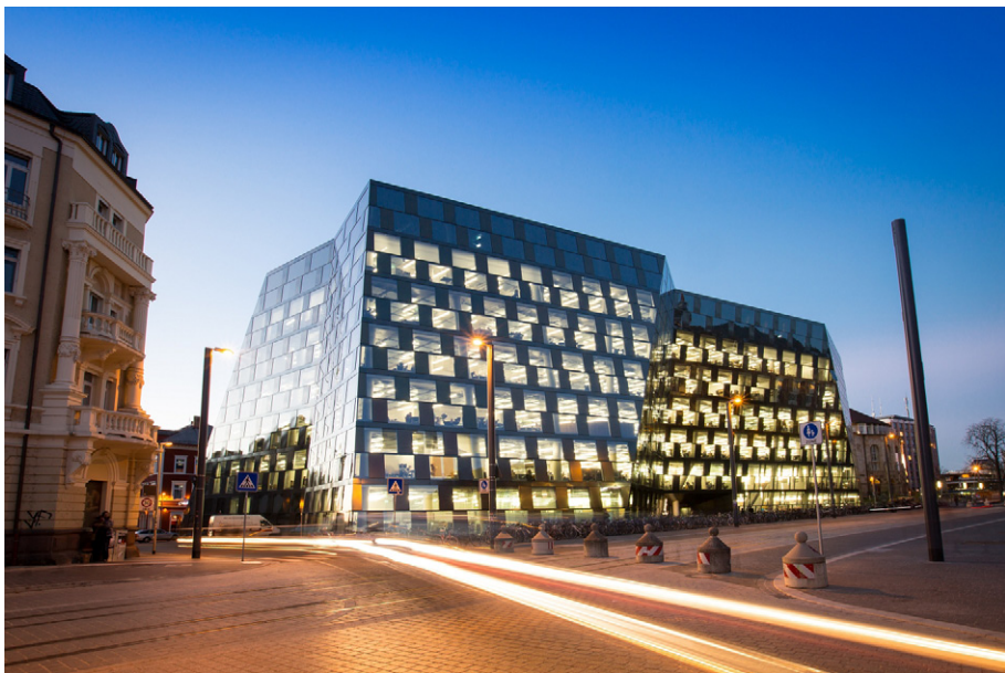
Exterior view by night © Sebastian Bender, Universitätsbibliothek Freiburg
