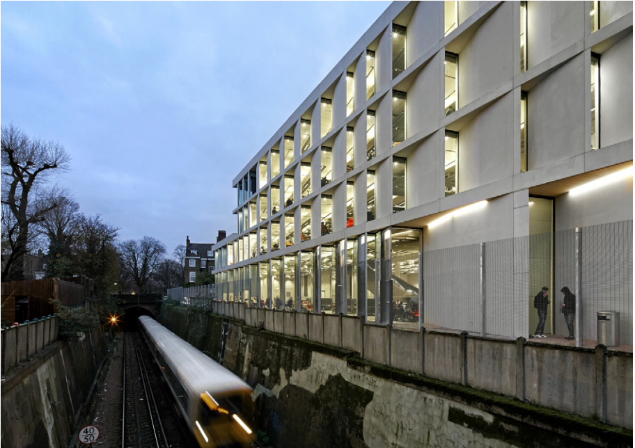
View of Library Facade © Hufton+Crow
