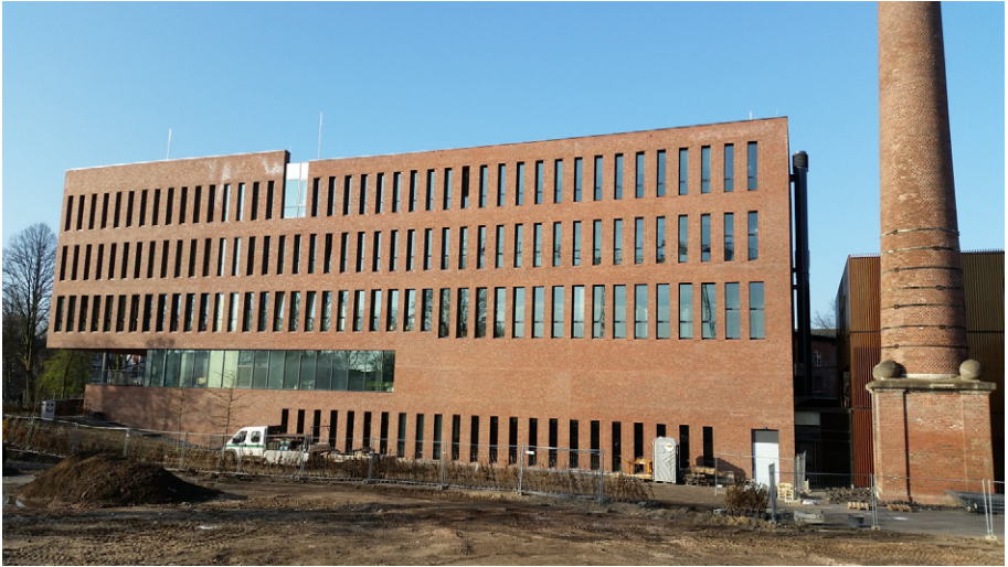
Northern Facade © Holger Wendt
