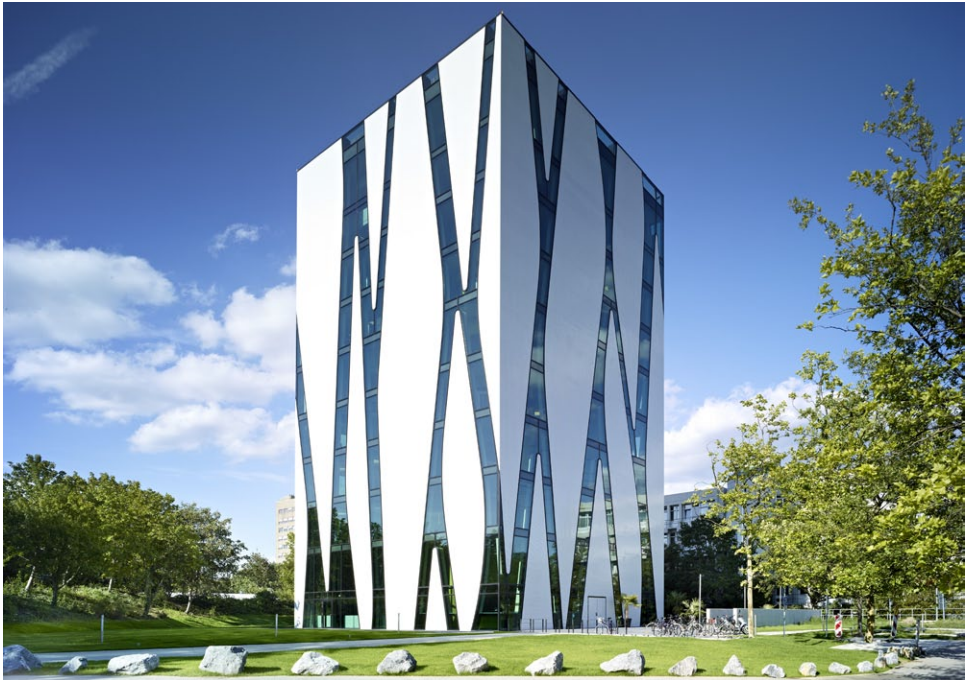
The Library Exterior HPP Architekten, Photographer: Ralph Richter
