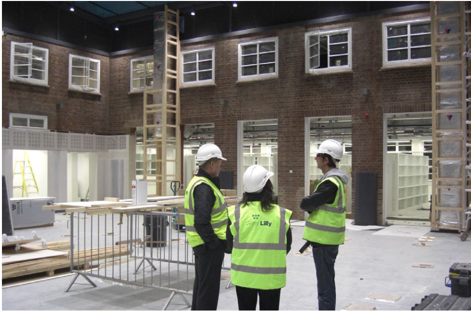
Dame Elizabeth Esteve-Coll Centre Atrium during construction © Kingston University
